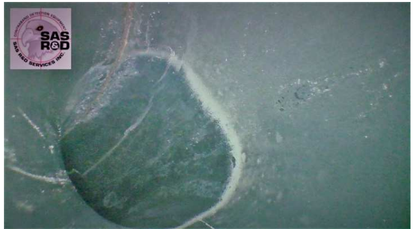
Inside Fuel Tank
